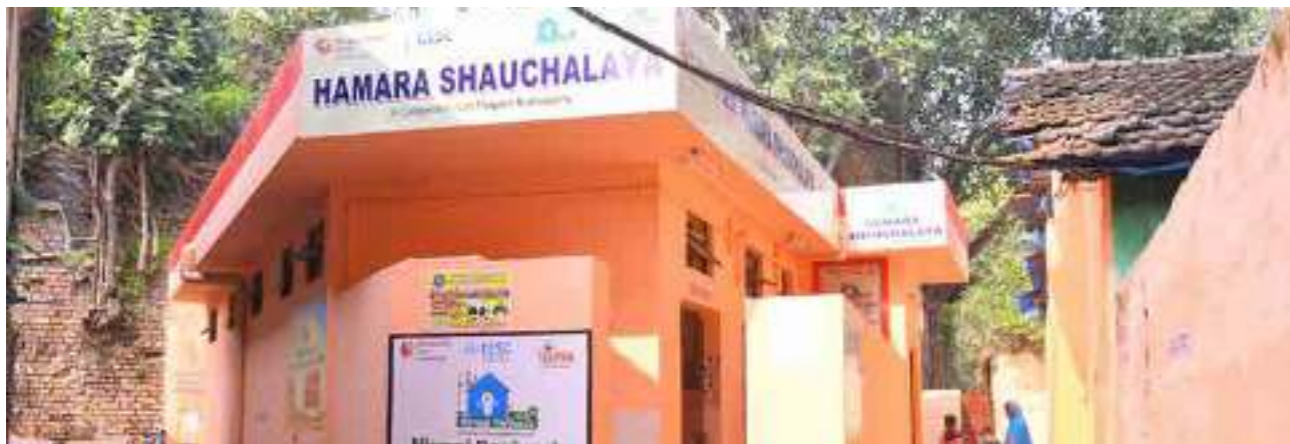
Establishment of pay and use toilets
