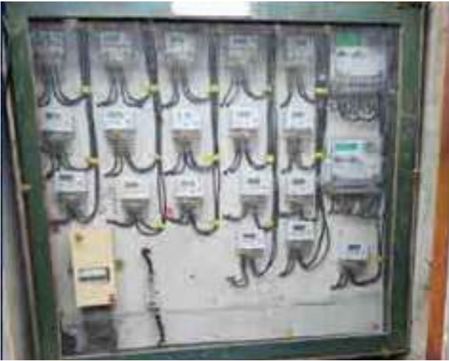
Renovation of Metre box
