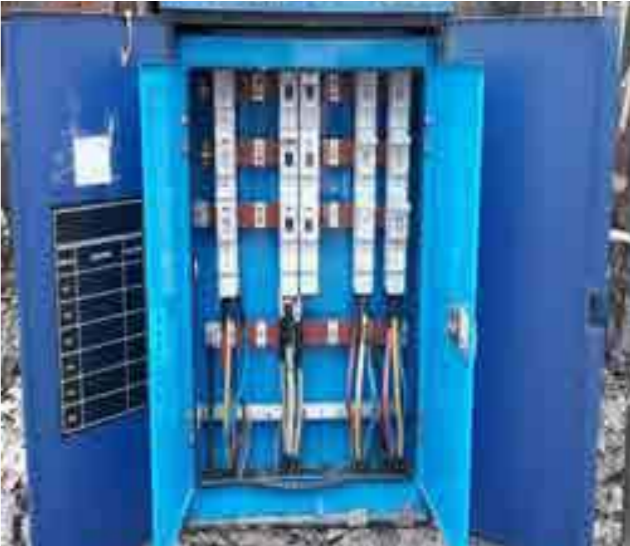
Installation of Anti-theft pillar box
