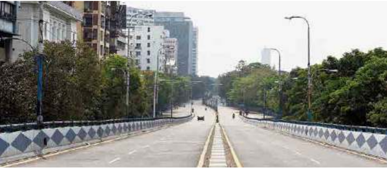
Maintenance of green verge from Park Street flyover to Hazra Crossing
