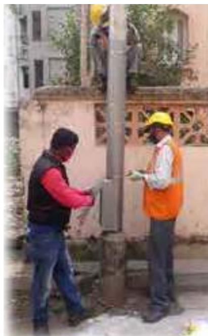
Timely maintenance of pillar boxes before monsoon
