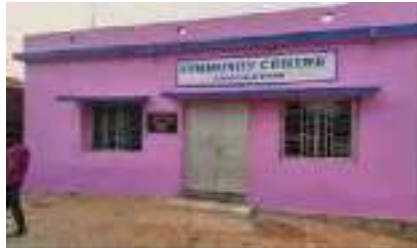
Construction of Community Centre
