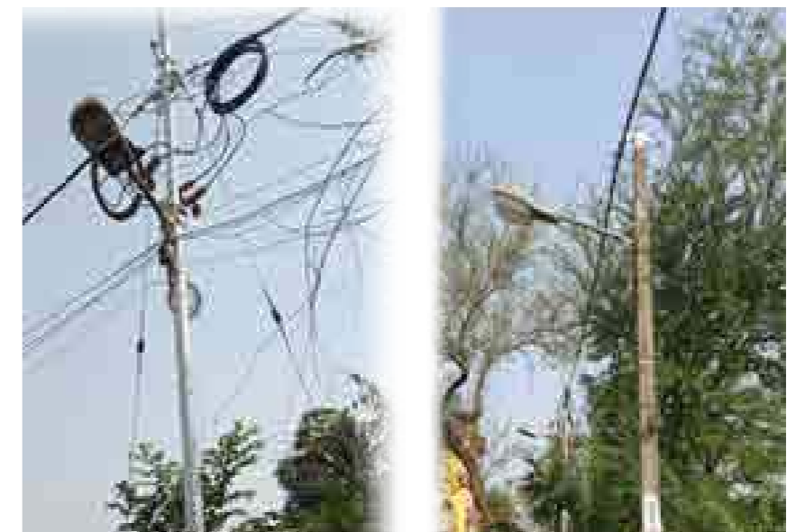
Installation of AB cables to replace bare overhead conductors
